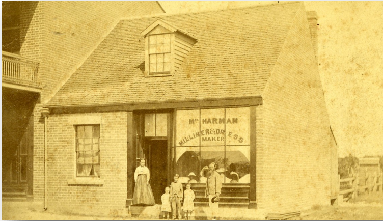
Original shop in Prince Street, Grafton. Presumed burnt down in the early 1880s and replaced with the current building. It is assumed that Elizabeth is on the left, William on the right and their three children
