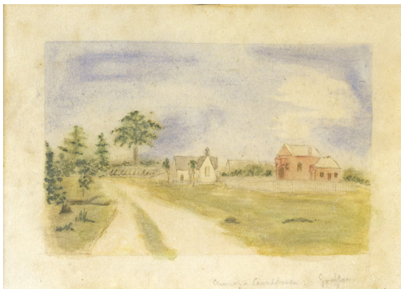
(Rose Selwyn, an early Clarence Valley artist, painted a watercolour sketch of that building in 1853).
